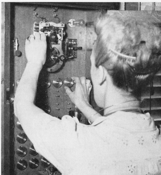
Helen McAvoy, chief telephone operator, upon receiving an alarm from a fire box, plugs in the disk which sends the alarm signal to the Repeater in Bldg. No. 48. Then the bells and horns sound.
